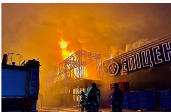
The aftermath of the shelling of a supermarket in Kherson, June 6, 2024.
