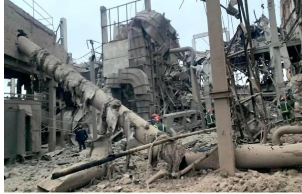
Okhtyrka TPP Source: Ukrinform
