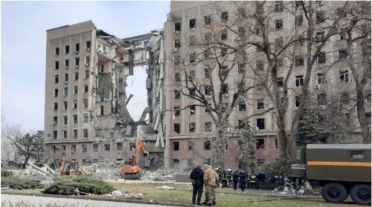
The destroyed building of the Mykolaiv Regional Council. March 29, 2022. Photo: Suspinne Mykolaiv
