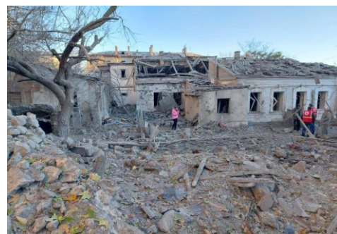
Destroyed lyceum and houses in Mykolajiv
